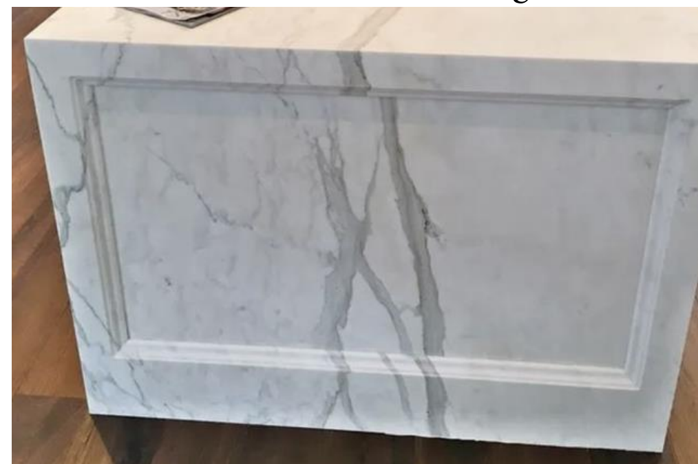
Panel Detail Behind Range Hood
